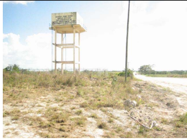
August Pine Ridge water tower, looking down road toward well
