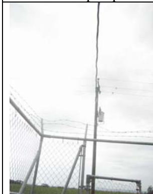
Transformer on power pole
